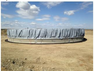
meaning installations are bolt, pin and clip free, resulting in 75% less parts than most other frac-water management alternatives.
